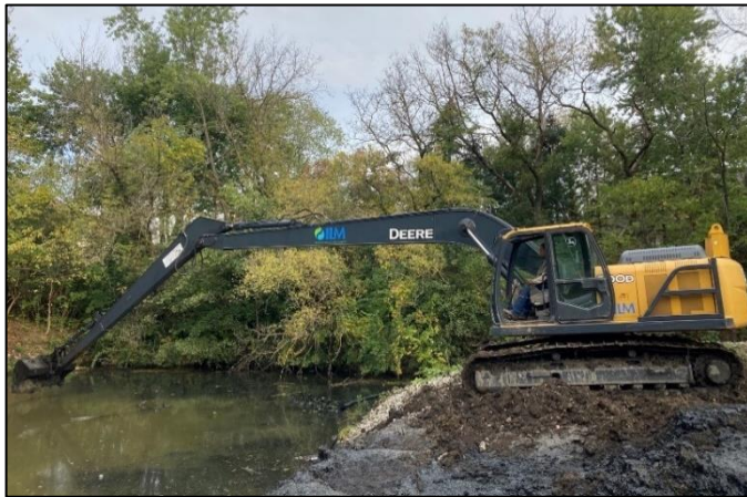
Photo 7. Mechanical sediment removal.
